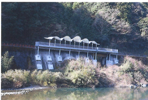
Special viewing platform Seiryu Miharashi Eki
